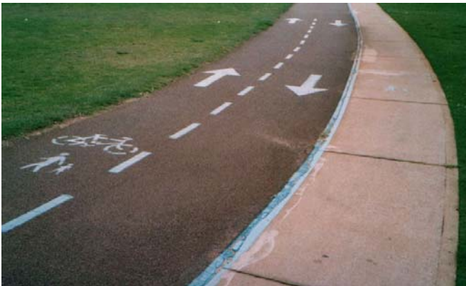
Markings on a shared pathway
