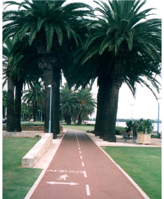
Markings on a shared path to indicate the presence of conflicting pedestrian movements
