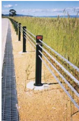
Figure 2. Pictures of deformable road infrastructure (Pictures from www.brifen.com and www.flexfence.com ).
